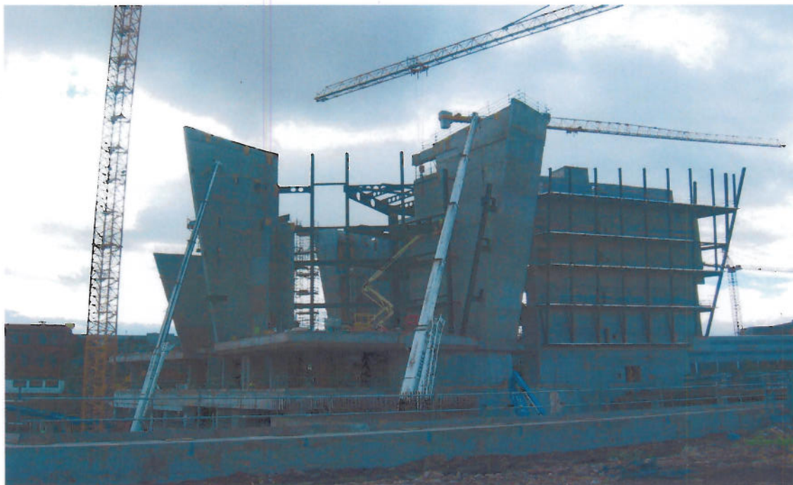
Photo 2: View from NW Corner of Site
