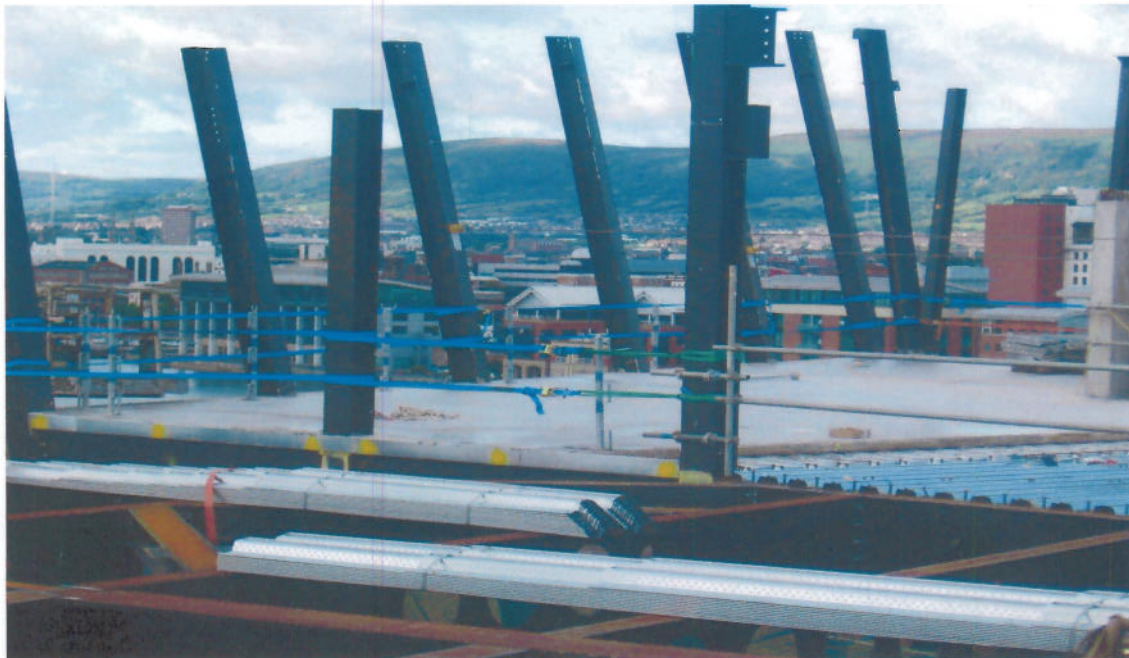
Photo 6: Hull 4 Level 5 Metal Decking & Concrete Floor
