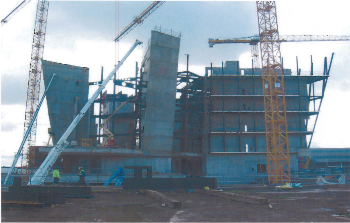
Photo 3: View of West Elevation
