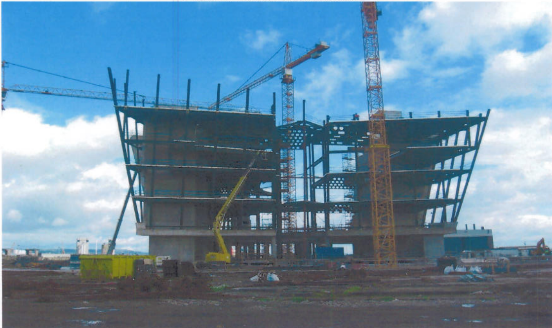
Photo 4: View of South Elevation
