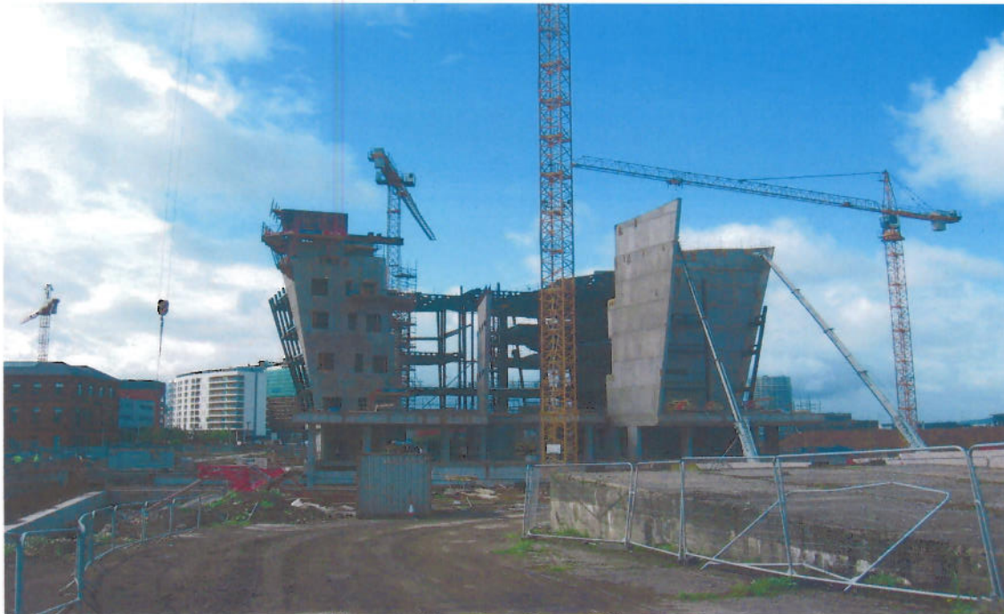
Photo 1: View from Top of Slipways
